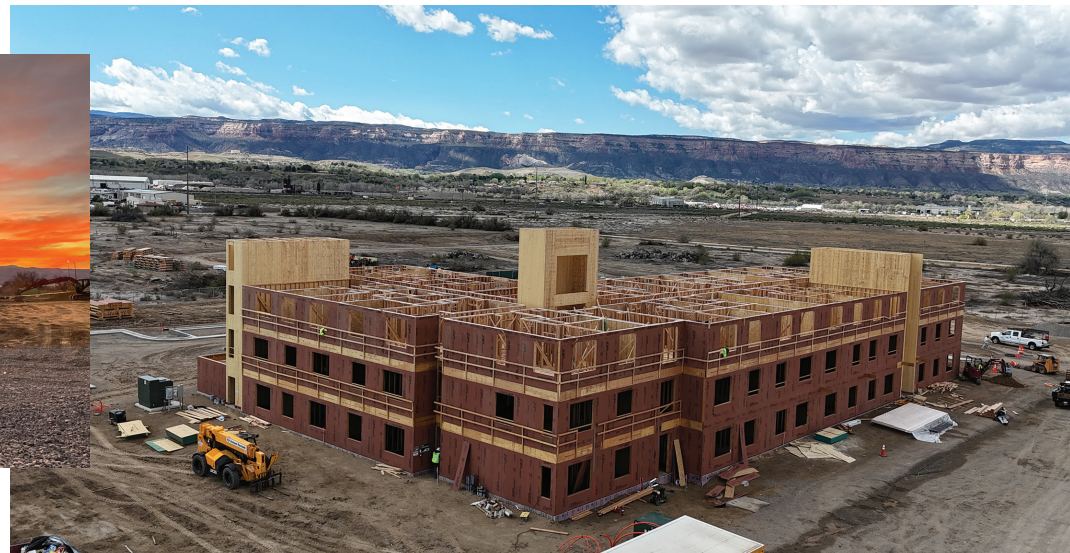
Third floor framing taken April 2, 2026
